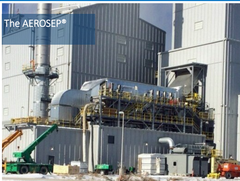
AEROSEP® Multi Stage Aerosol Separation System installed in a urea granulation plant to control particulates and ammonia vapors. Gas flow exceeds 500,00 M3/hr.
