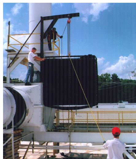
B-GON® Mist Eliminator pad used to control sulfuric acid mist generated from lead-acid battery production
