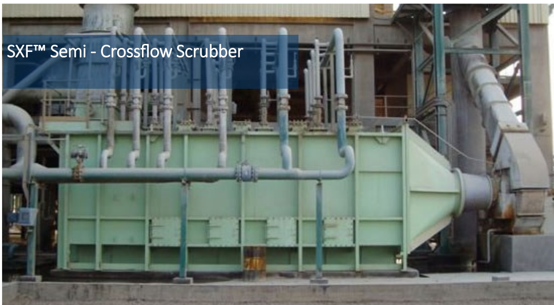
SXF™ Scrubber installed in phosphoric acid plant controlling fluorine vapors
